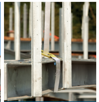
Industrial hall construction
