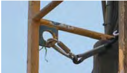
Anchorage Point – Your platform will have a designated harness anchor point
