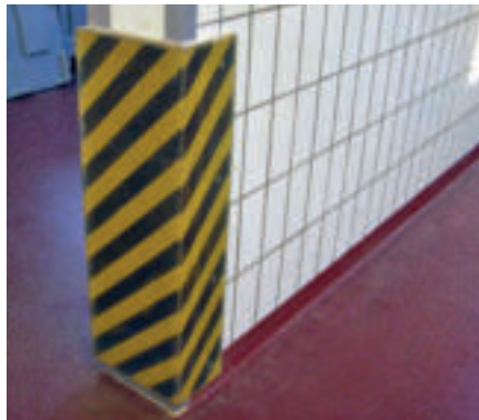
secutex impact protection (black/yellow paint coating on perforated sheet) reliably protects walls and corners when impacted by forklifts and pallet trolleys.
